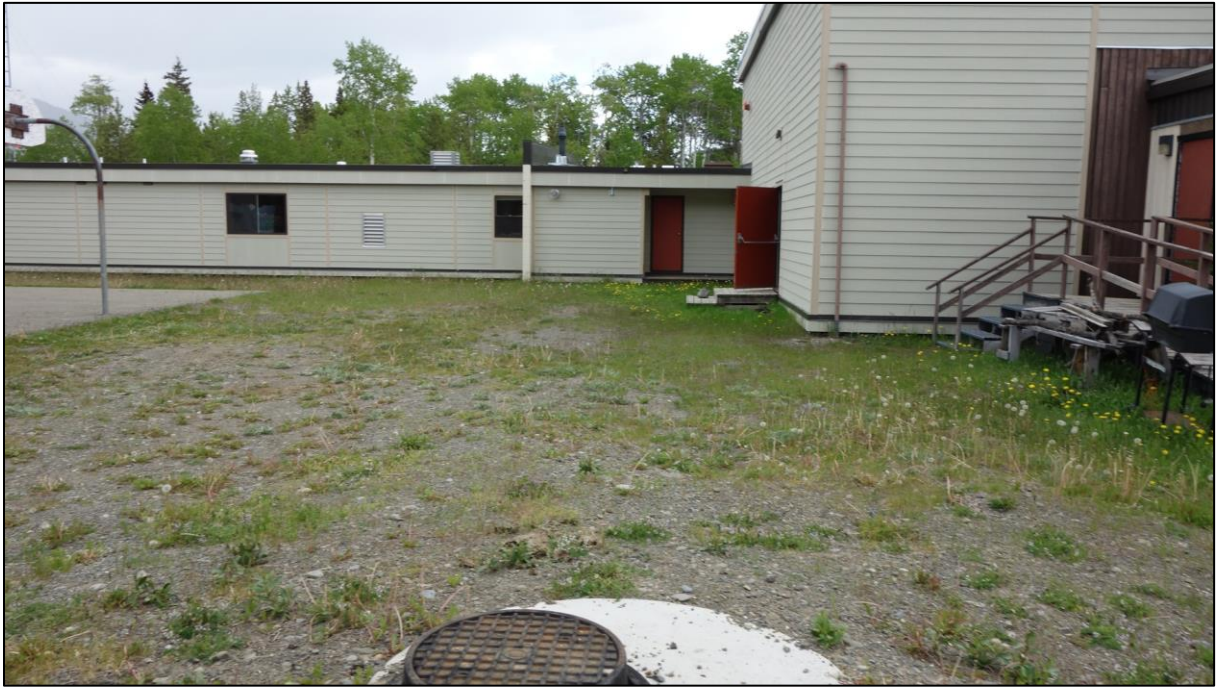
Photograph 31: Vicinity of UST at Naghtaneqed School, located adjacent to the west of Lohbiee 3, looking east
