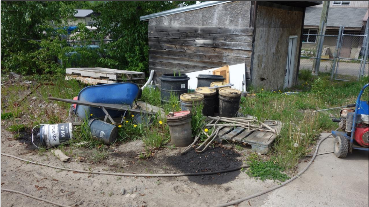
Photograph 6: Stains and waste oil adjacent to pressure washer on Enterprise Works Yard fuel pump pad, looking southwest
