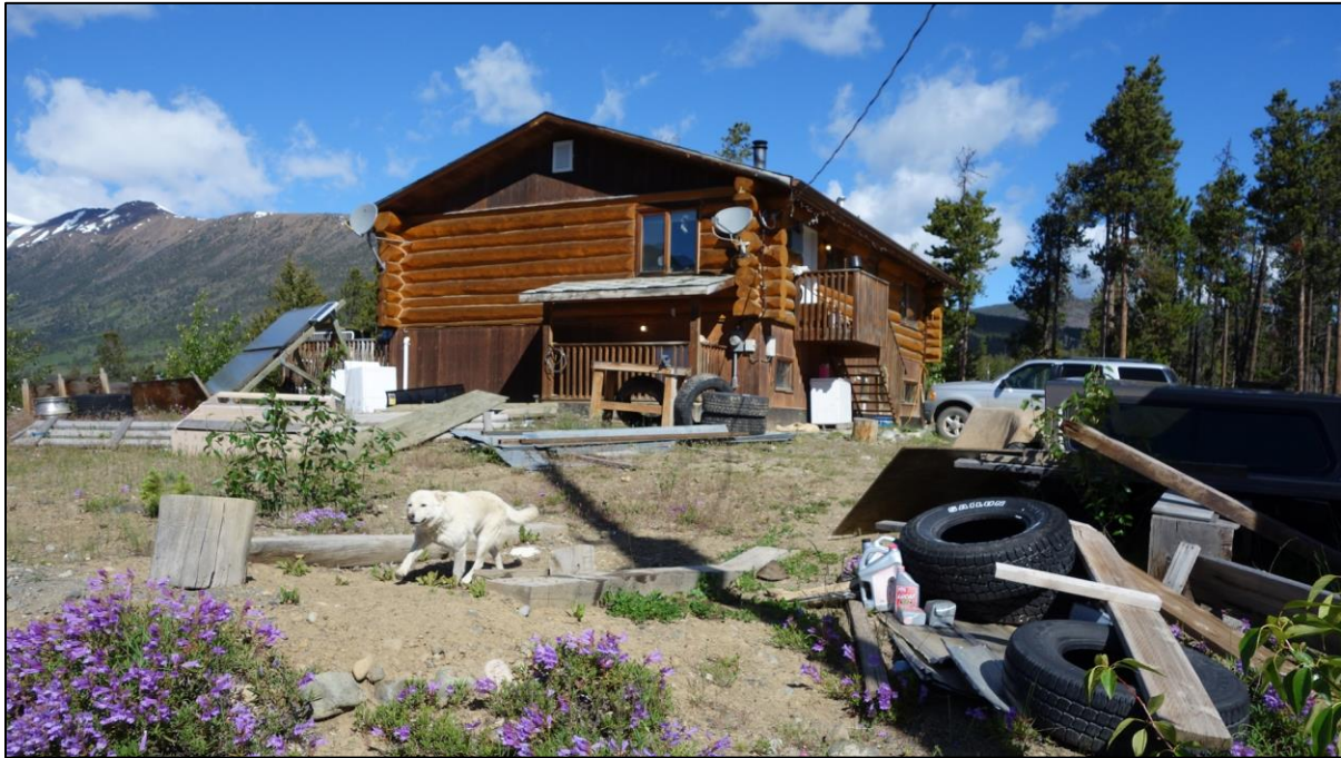
Photograph 25: Kerry Billy/Bruce and Darleen William residence, located on the northwest portion of Lohbiee 3, looking northwest
